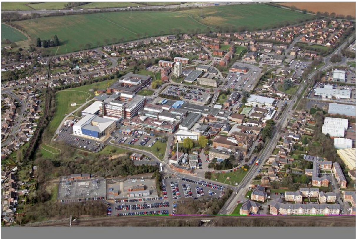
Kettering General Hospital, Rothwell Road, Kettering
